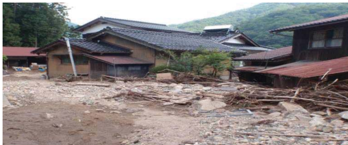
Fig. 2 The precipitation in Tuwano-Cho on 28 th July in 2013 and its avalanche of rock and earth
